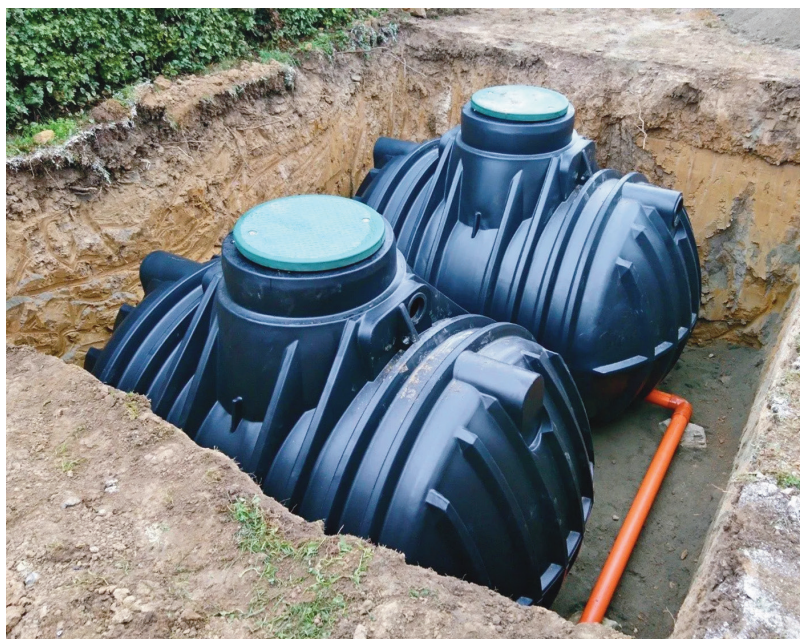
FIGURE 02: Prefabricated septic tank during underground installation. Source: Bowen's Septic Tank.
