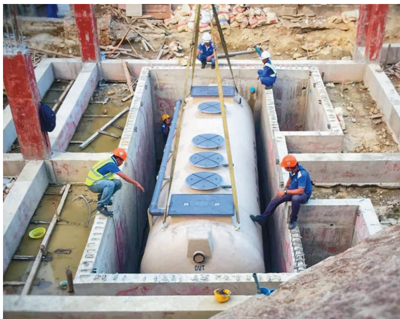
FIGURE 09: Johkasou Tank during installation. Source: Charm Limited.
