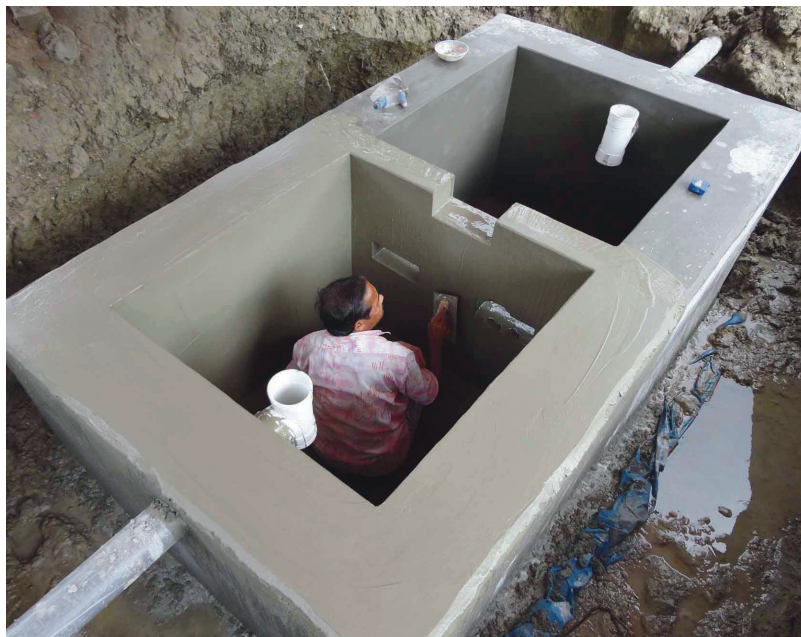
FIGURE 01: Two-chamber septic tank during construction. Source: Healthabitat.
