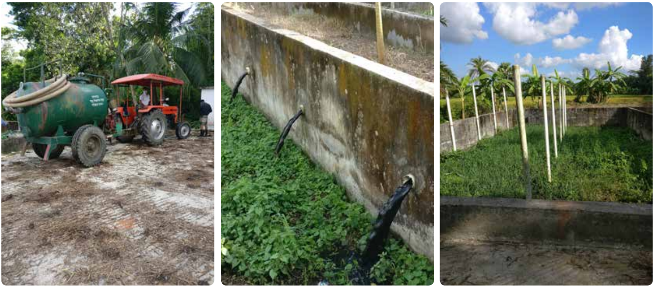
FIGURE 2: Lakshmipur – Desludging Vehicle and Planted Drying Bed
