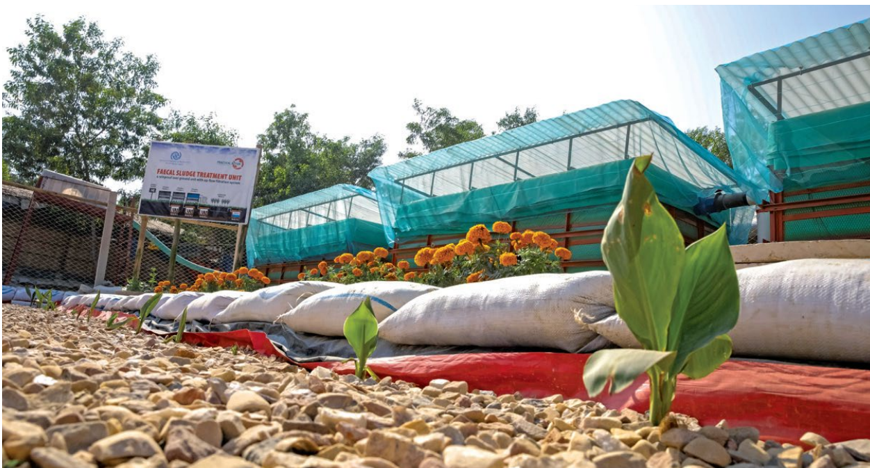
Figure 19: Constructed wetland of the FSTP
